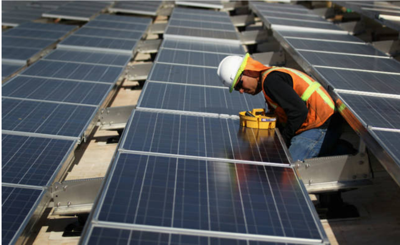
A workman installs solar panels in Colorado. Credit: John Moore/Getty Images
